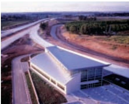
The state-of-the-art operations centre for the Cross Israel Highway
