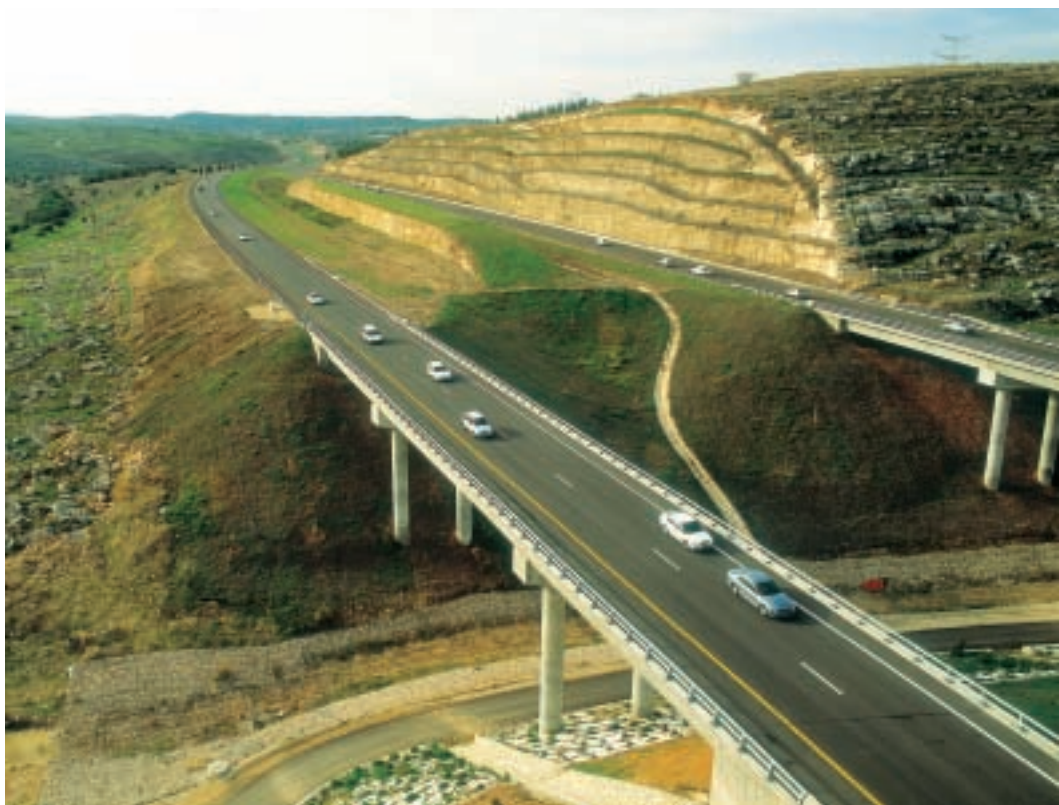
Above: Cross Israel Highway bridges at the Natuf valley near Shoham Previous page: The Cross Israel Highway at the Ben-Shemen Interchange near Tel Aviv
