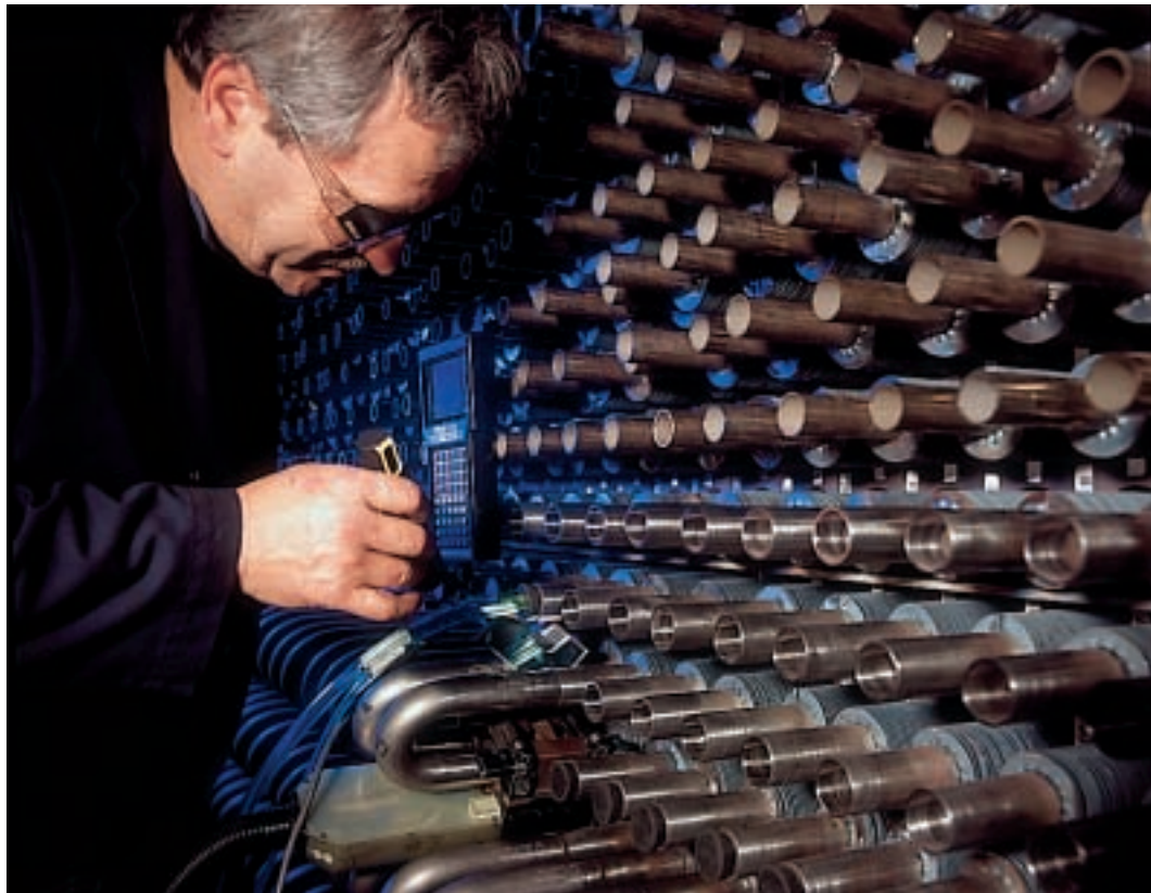
Pressure parts being installed during the final assembly of an OTSG module. Each tube connection is welded using IST's highly specialized orbital welding system.
